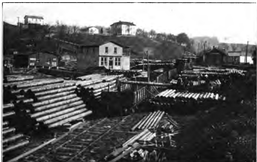
PLATE II (a).—Handling Pipe at Tollgate for a large natural gas line for this region.
